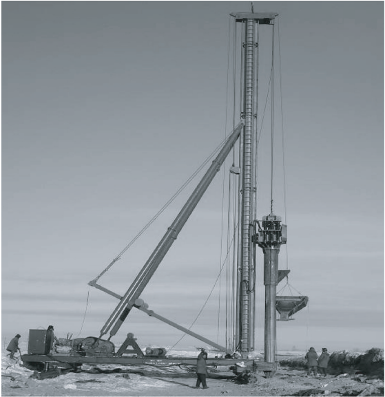
图 1 土工织物散体桩施工 Fig.1 Construction of the discrete material pile
